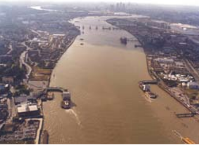
From Woolwich looking West we see the inner marker beyond which river defences may not be compromised. ©Thames Gateway, Communities & Local Government
