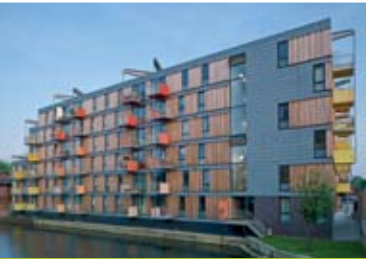
■■■ Adelaide Wharf, London. Winner, Housing Design Awards 2008. Architect - Allford Hall Monaghan Morris ©Tim Crocker
