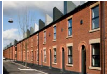
■■■ Chimney Pot Park, Manchester. RIBA Northwest Award 2008 and shortlisted for RIBA Stirling Prize, in association with The Architects' Journal. Architects - Shed KM with Urban Splash © Morley Von Sternberg
