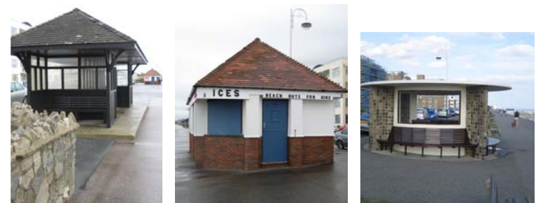
Above, existing seafront structures to be replaced
