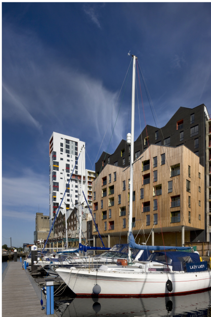
Scheme: The Mill, Ipswich Architects and location: John Lyall Architects, London Photo credit: Morley Von Sternberg
