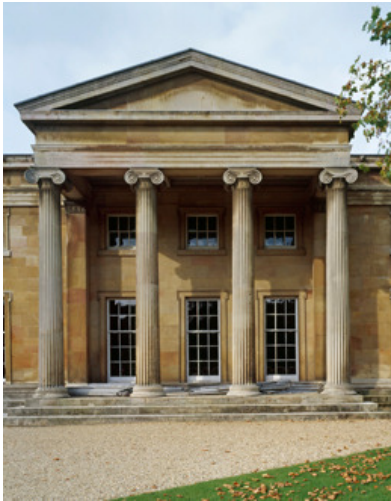
Scheme: Downing College, Cambridge Architects and location: Caruso St John Architects, London Photo credit: Ioana Marinescu
