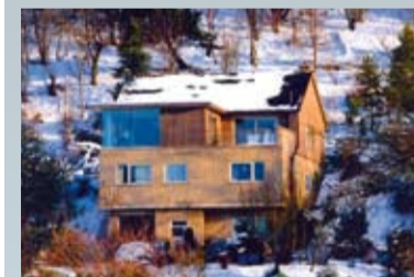
Rooftop extension at private house, near Matlock Architects: Evans Vettori Architects Photography: Martine Hamilton Knight
