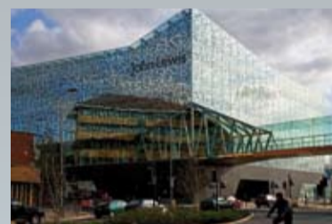
John Lewis Department Store and Cineplex, Leicester Architect: Foreign Office Architects Photography: Peter Jeffree/Helene Binet/Satoru Mishima
