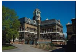
Abbey Mills Pumping Station © Thames Water
