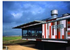
RIBA Awards 2007 RSPB Rainham Marshes Nature Reserve van Heyningen & Howard Architects © James Brittain
