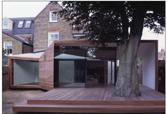
Wrap House (above) by Alison Brooks Architects has been shortlisted for both The Stephen Lawrence Prize and The Manser Medal. The Stephen Lawrence Prize is sponsored by the Goldschmied Trust and rewards the best examples of projects with a construction budget of less than £1 million.
