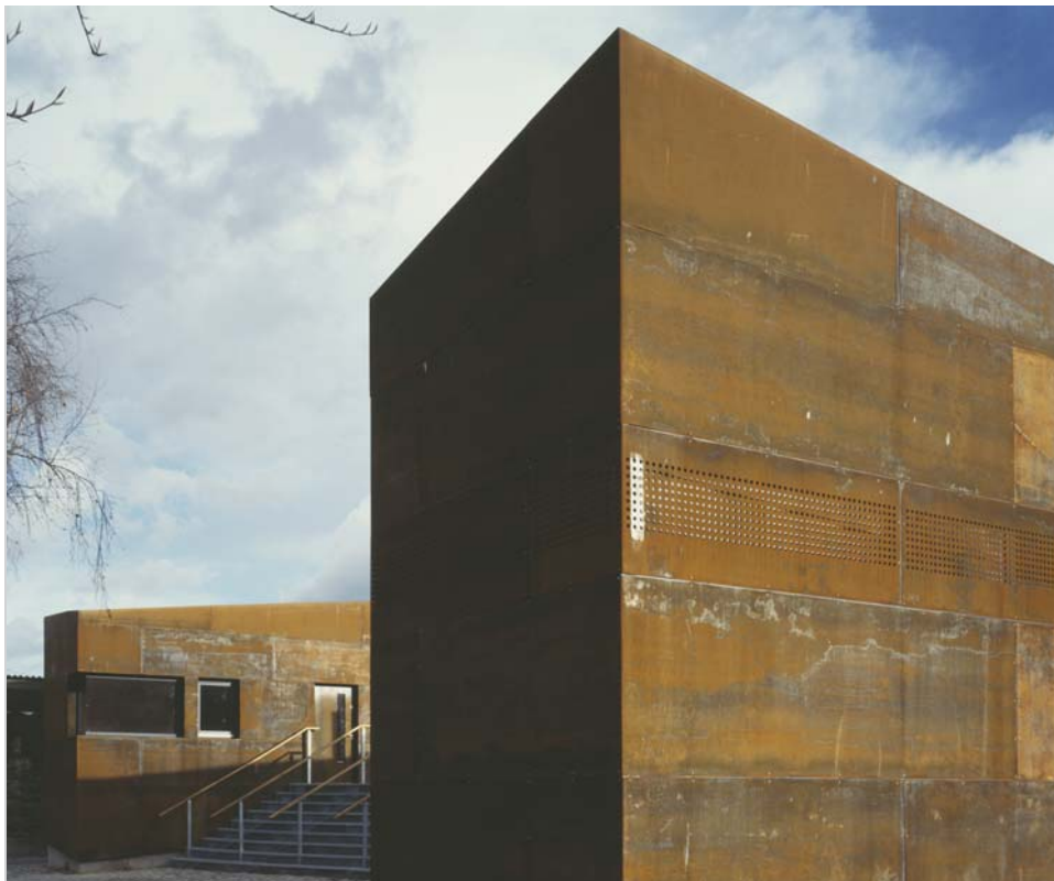
Cremorne Riverside Centre by Sarah Wigglesworth Architects Photograph: Ioana Marinescu
