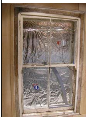
6. As Option 5, with low emissivity plastic film fixed to the window facing side of the blind U value 1.8 Heat loss reduced by 61%
