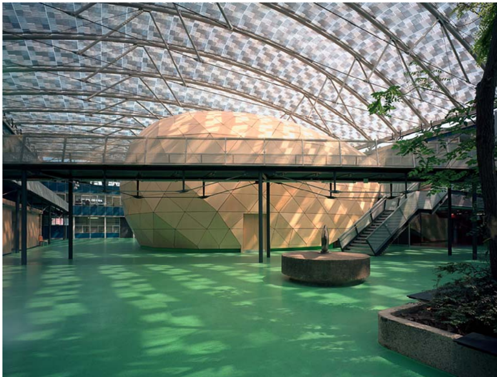
Illustration 01; Kingsdale school ETFE 'variable skin' roof & plywood auditorium; Photo: Alex de Rijke
