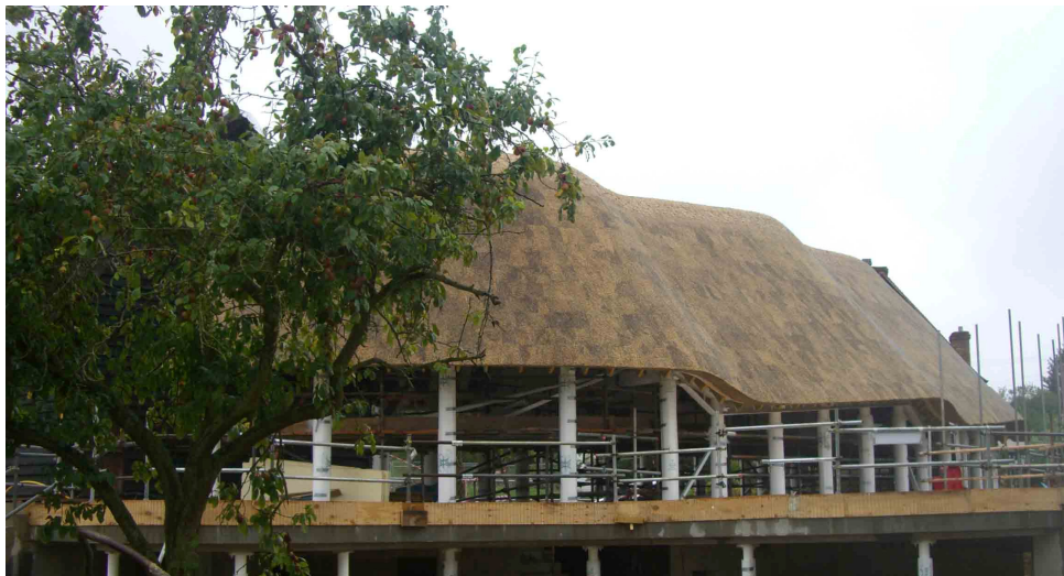
Illustration 3: The pool house on site.
