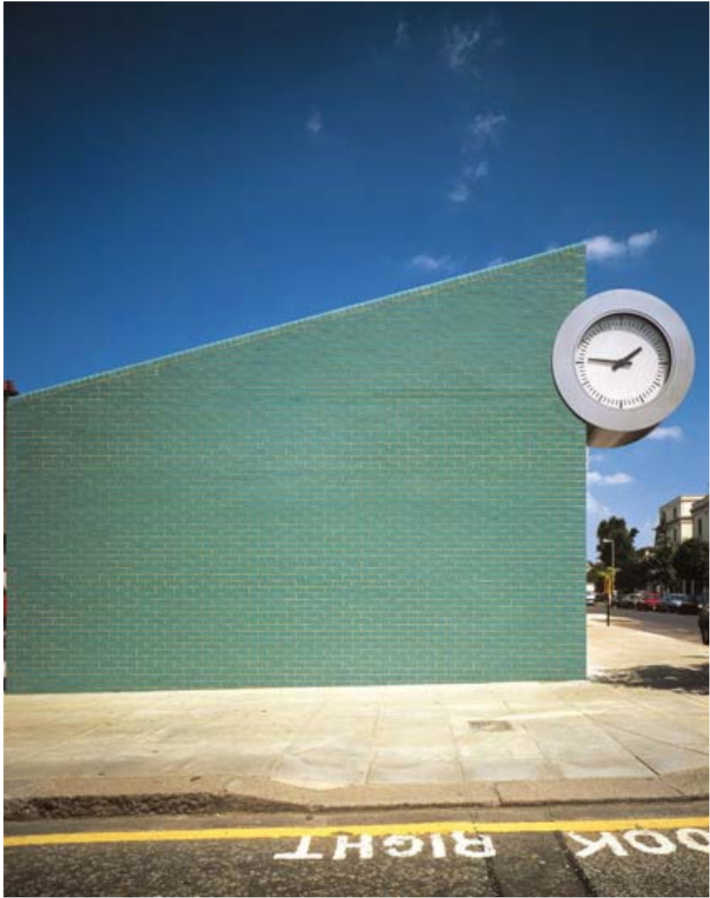
Illustration 9: CZWG, public lavatories, Westbourne Grove, detail showing wall
