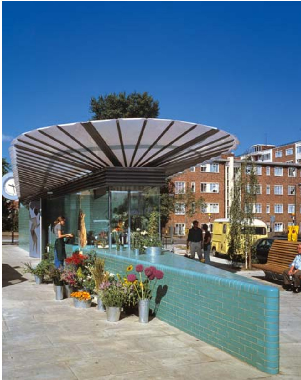
Illustration 8: CZWG, public lavatories, Westbourne Grove
