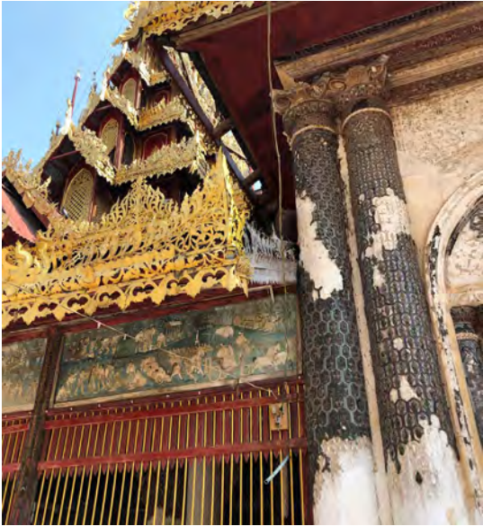
Junction on the north facade of the Hna-Kyeik-Shit-Su Shrine showing the loss of external finishes on the relief columns
