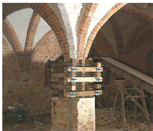
Pre-reunification column and vault repairs in the Ratskeller used hard new brick and cement rendering (rear of the image). The repairs under Purcell's direction conserved brick ribs and lime-washed the vaults are in the foreground. The 1890's brick casing to the column was repointed and limewashed too.
