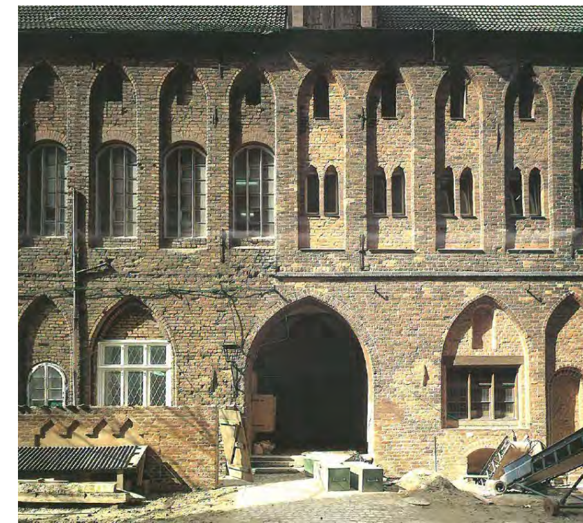
On the ground floor of the restored facade (right), pre-reunification work had replaced carved baroque or earlier mullion-and-transom windows with speculative reconstructions. The facade on the left retains its building biography, and was repairable.
