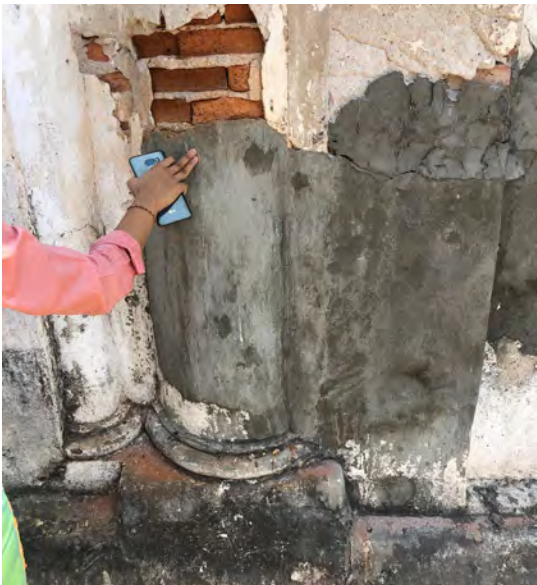
Image of unsuitable concrete render repairs on the south gable wall of Dipinkara Shrine
