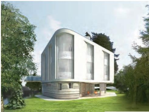
damage to the exterior of the building. However, flood resistance may only be effective with shallow flood depths or high-quality reinforced construction that can resist hydrostatic pressures<sup>2</sup> or impact of debris. The stilts upon which buildings are elevated must be capable of resisting flood waters, scour to the foundations and the impact of flood-borne debris in order to provide effective protection and stability.
