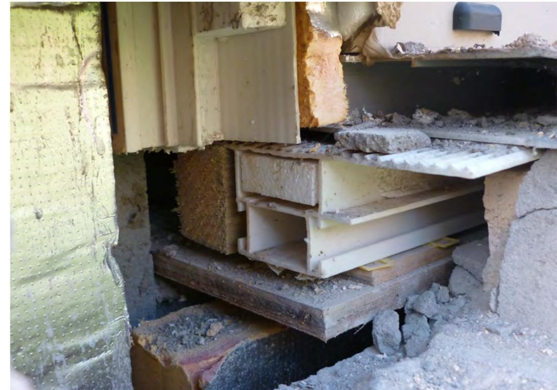
When design and construction are separated by contract, oversight of quality control and independent scrutiny are jeopardised. External wall cavity from a recent housing project reveals multiple defects, including non-fire rated materials & discontinuous components.
