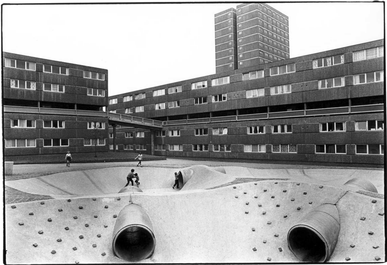
Photograph by Tony Ray-Jones of housing constructed using the YDG (Yorkshire Development Group) system. (RIBA pix ref no: RIBA2760-20)
