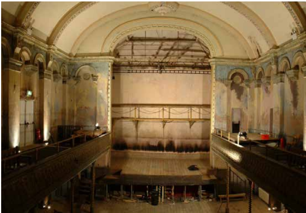
Auditorium from back of balcony 2003 © Wilton's Music Hall
