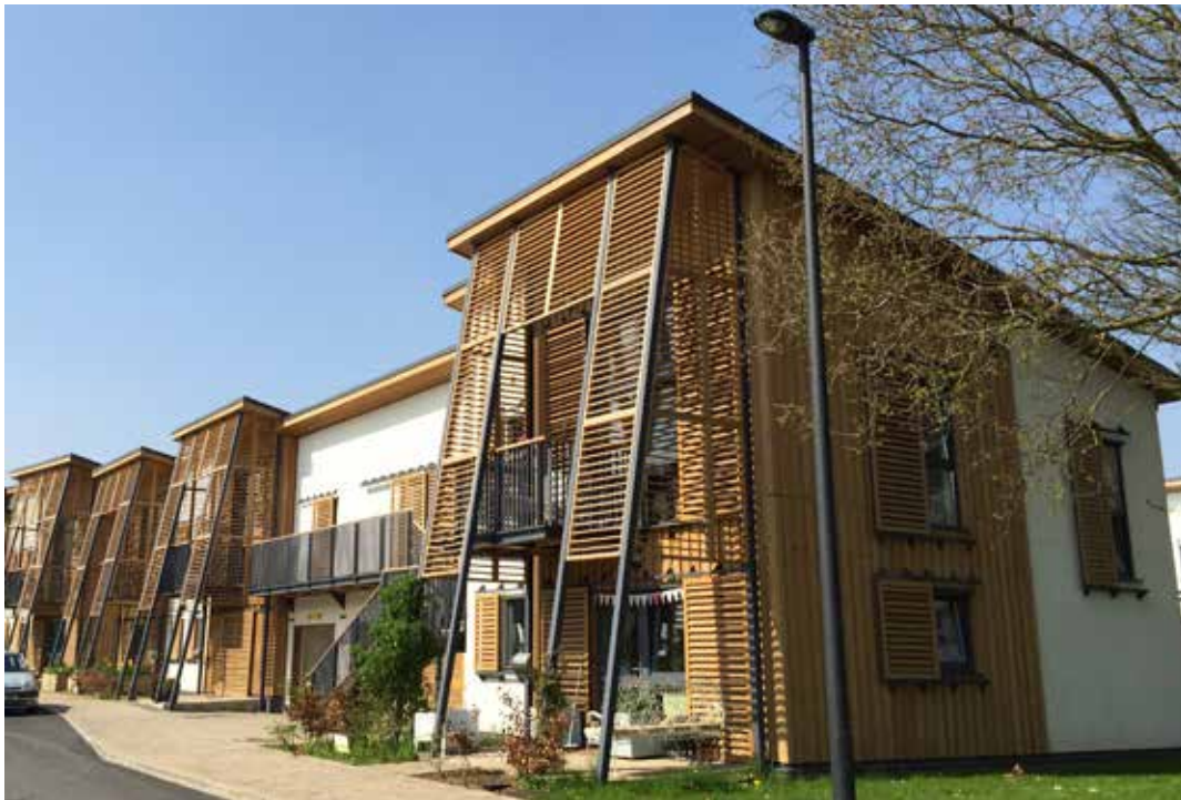
Hanham Hall Project © BSRIA Ltd
