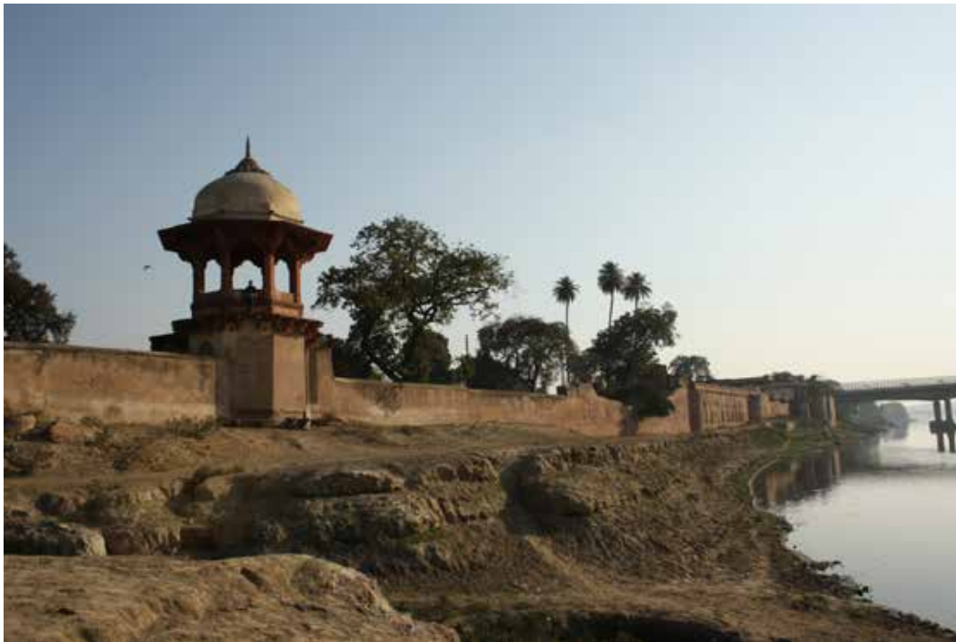
Remnants of 17th century Mughal gardens continue to line the Agra waterfront © Aylin Orbasli
