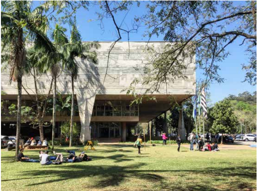
Façade of the Faculty of Architecture & Urbanism at the University of Sao Paulo (FAU-USP) © Raphael Selby
