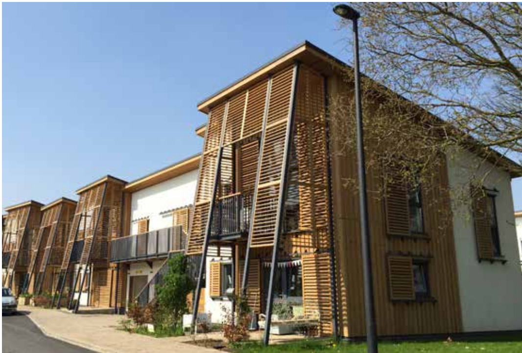
Hanham Hall Project © BSRIA Ltd
