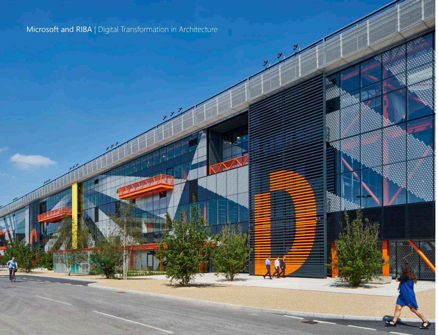
For the Here East Broadcast Centre Hawkins\Brown developed a unique 'dazzle pattern' facade, which was achieved by printing a ceramic frit onto curtain wall glazing. By using generative design software Hawkins\Brown were able to optioneer for the client, the pattern at building, human and micro scales. Here, the client and design team could accurately preview the aesthetic outcome but also, ensure that the frit performs technically. © Hawkins\Brown Architects; CGI artists The Neighbourhood; photographer GG Archard
